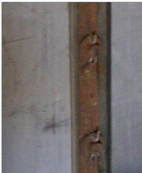
ABOVE: Cast iron chain installed in 2006 is already corroded and needs to be replaced (photographed in 2010).
